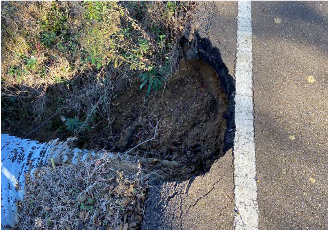
Above: Culvert/erosion at Stout Road, west of Calhoun Station Parkway.
